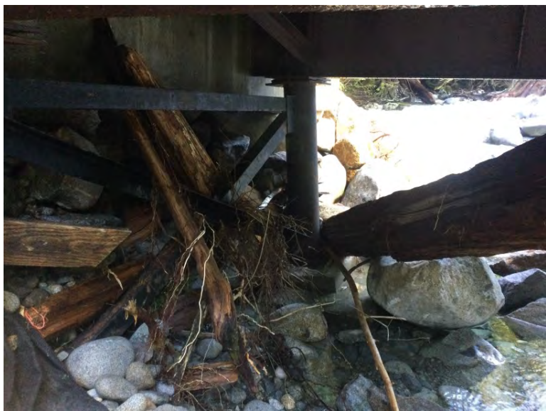
Upstream woods pipe column condition
