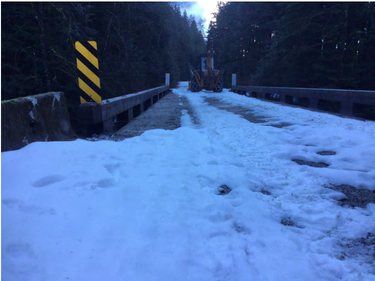
Upstream woods end deck lower in elevation
