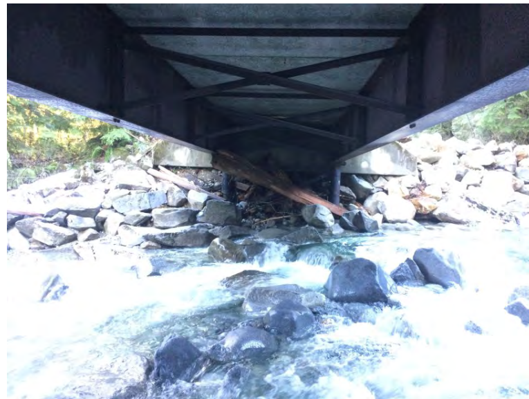
Right Bank Abutment when facing downstream
