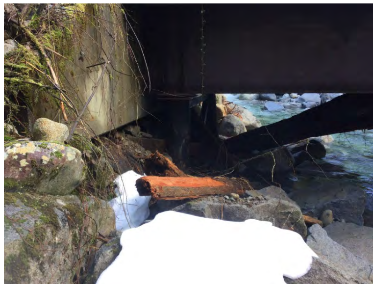
Right Bank Abutment when facing downstream
