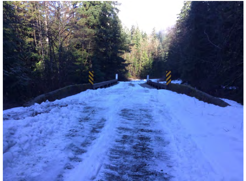
Approach from Left Bank when facing downstream
