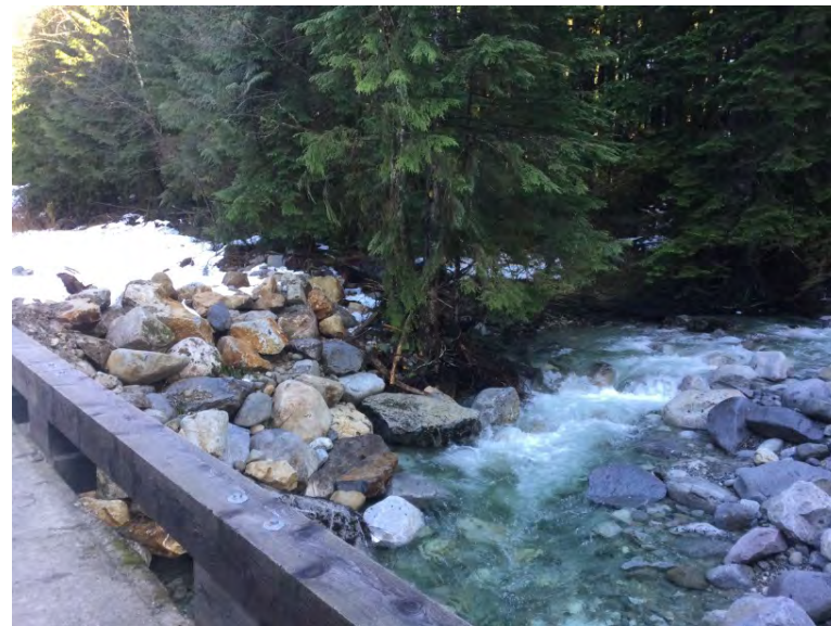
Upstream woods abutment
